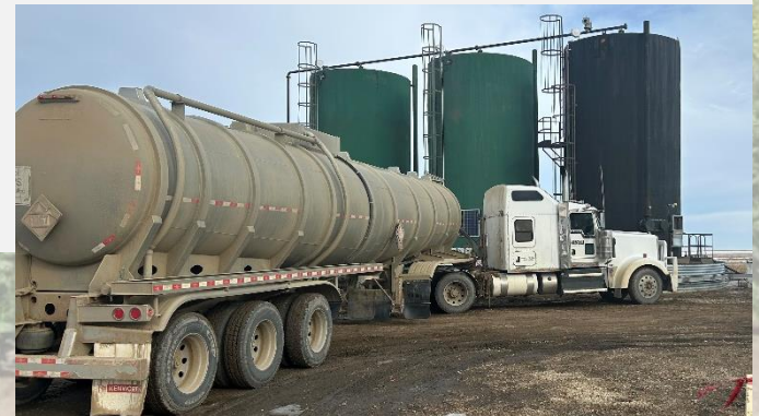
Shipping oil from the battery April 7, 2023
